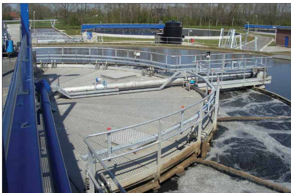
Figure 1: The modeled clarifier tank in the wastewater treatment facility. Photo courtesy of Witteveen+Bos.
