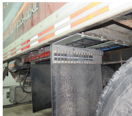
FIGURE 2. Top: Galvanic corrosion damage induced on a multimaterial overlap assembly made of a carbon-fiber-reinforced polymer (CFRP) and a 6000 series aluminum alloy after one year of in-service exposure on a vehicle. Bottom: Typical mounting of samples on a vehicle for in-service exposure testing.
