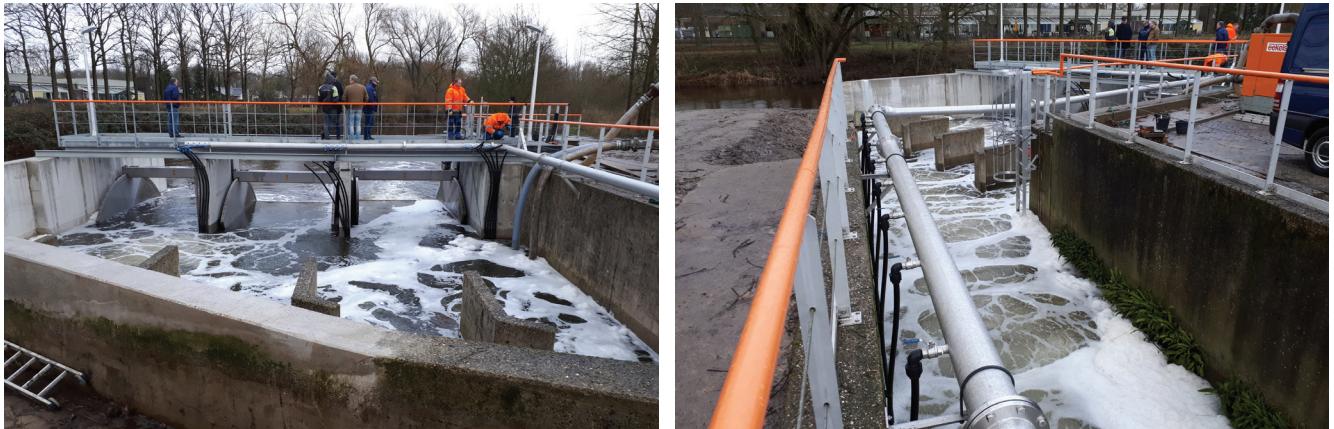
FIGURE 7. The aeration channel of the Eindhoven Wastewater Treatment Plant in full operation as it improves the oxygen quality of the effluent before reentering the Dommel. Left: View of the adjustable dam at the outlet of the aeration channel. Right: View of the aeration channel from the inlet.
