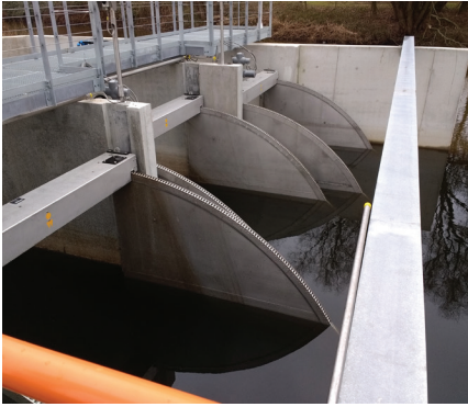
FIGURE 3. View of the adjustable dam at the outlet of the aeration channel.
