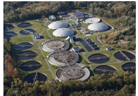
FIGURE 1. Aerial view of the Eindhoven Wastewater Treatment Plant.
