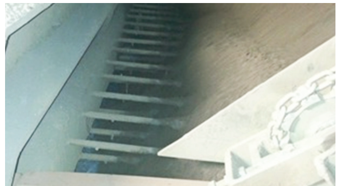
FIGURE 5. Sinter plant feeding system in operation with two rows of horizontal permeability bars.
