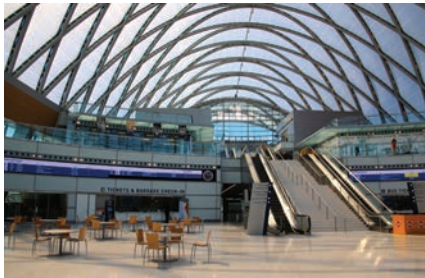
FIGURE 5. Top: ARTIC with radiant heating system installed, prior to the actual flooring being laid. Bottom: End result of the inside of ARTIC.
