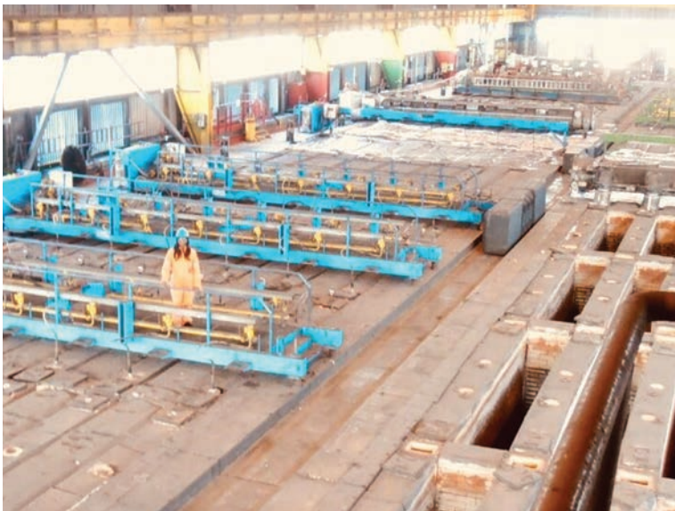
FIGURE 1 Anode baking furnace at Aluchemie.
