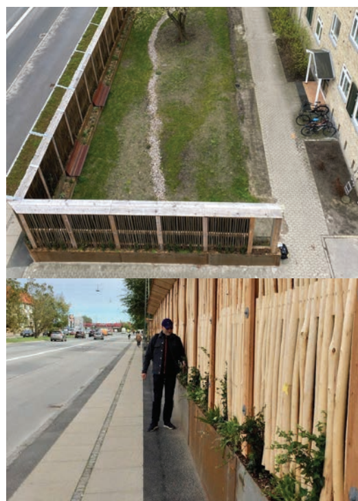
FIGURE 9 An overhead view of the completed structure and a street-side view of the urban green screen.
