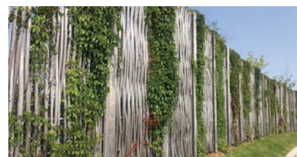
FIGURE 4 A Pilebyg noise barrier along a Danish highway.
