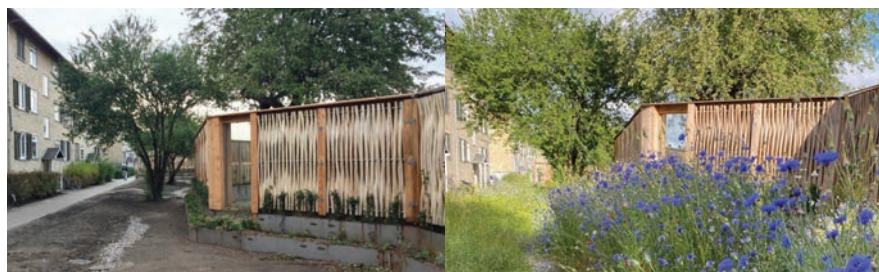
FIGURE 8 A section of the completed urban green screen in 2019 (left) and 2020. Note the vertical glass window and the emergence of native plant life between the screen and buildings.
